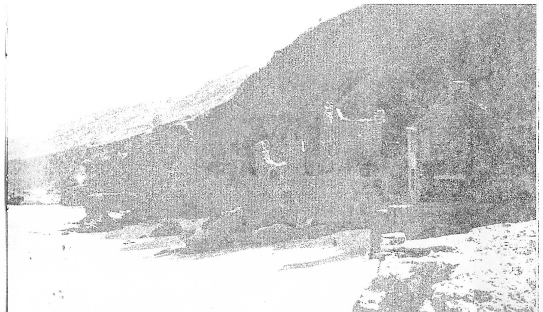
10 The ruined village at Hallsands on the S Devon coast, England. The village was built on a coastal ledge (an emerged shore platform) 4-5 m above mean sea level. A broad shingle beach formerly stood in front of it, but removal of shingle resulted in accentuated erosion at the cliff base. (C. T. Bird)
