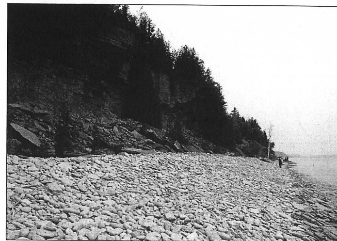
Figure 13.7 Erosion of shale at the cliff toe leading to undercutting and failure of blocks of relatively resistant sandy dolomite, Cape Dundas, Georgian Bay, Ontario. The shale is one of the lower units in the Niagara Escarpment. Note the rectangular jointing pattern in the overlying rocks which controls the size of the failure blocks.
