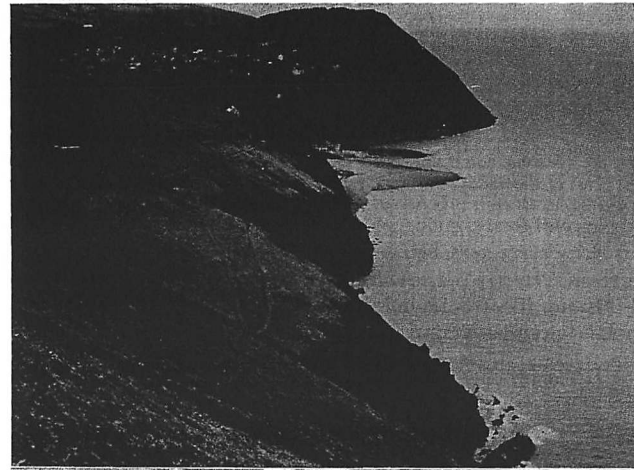
FIG. 67. Slope-over-wall cliffs near Lynmouth, southwest England.
